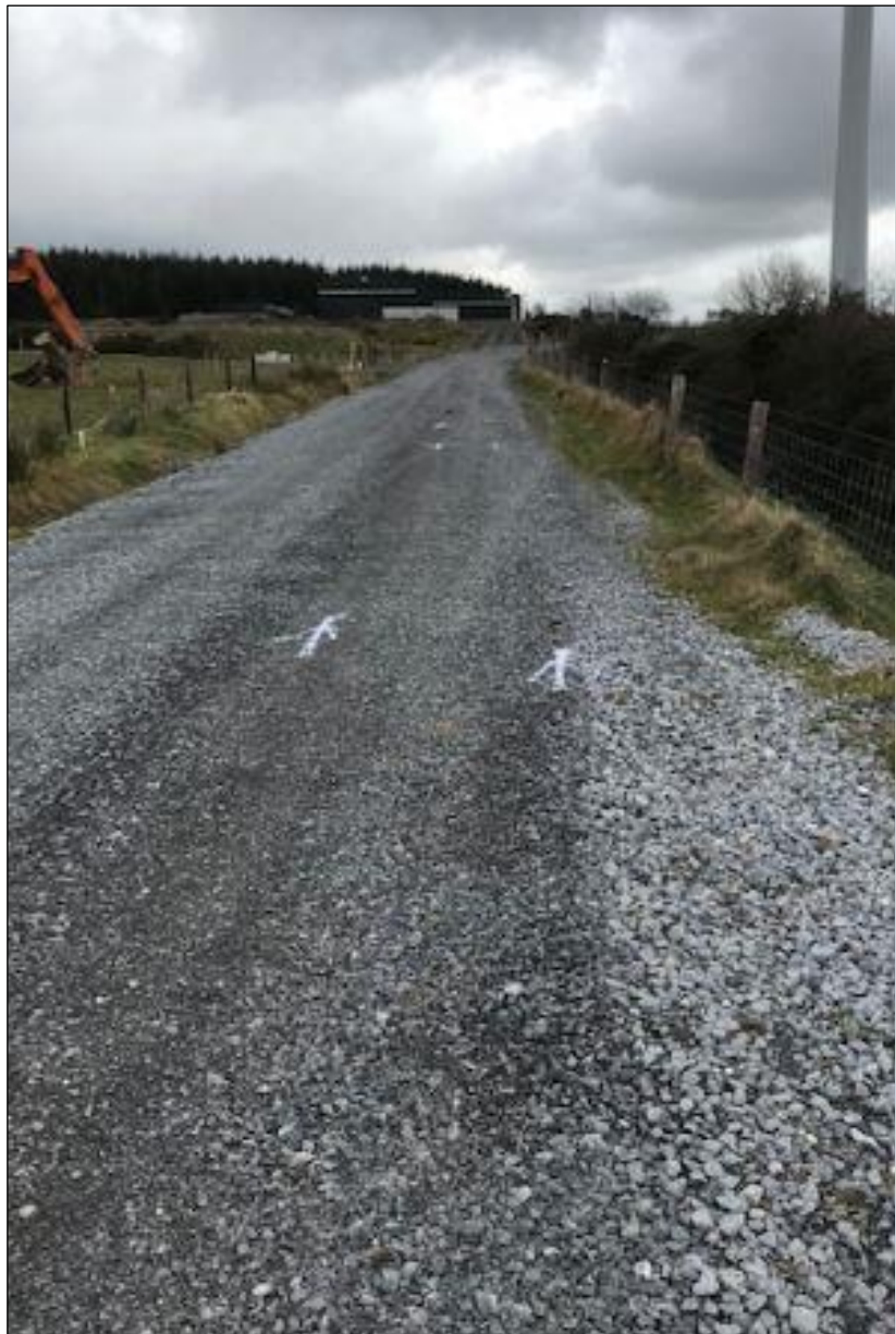
Figure 3.6: Typical On-Site Access Track
