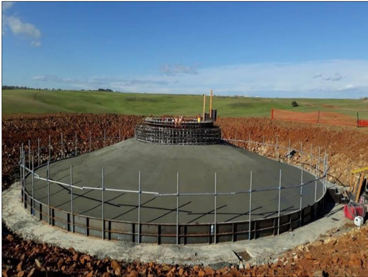
Figure 3.5: Typical Turbine Foundation
